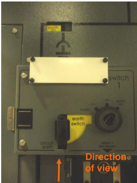
4.20 RSW1 Service position Earth selected Earth ON
