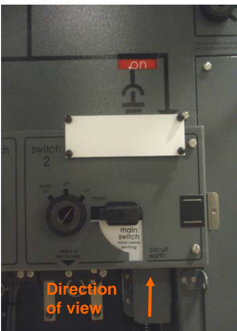
4.8 RSW2 Service position Main selected Main ON
