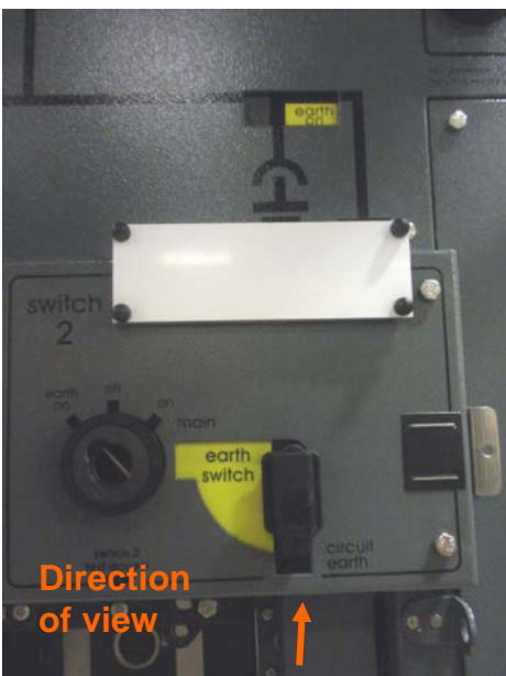
4.20 RSW1 Service position Earth selected Earth ON
