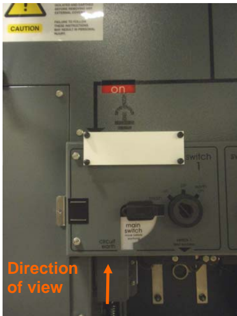
4.8 RSW2 Service position Main selected Main ON
