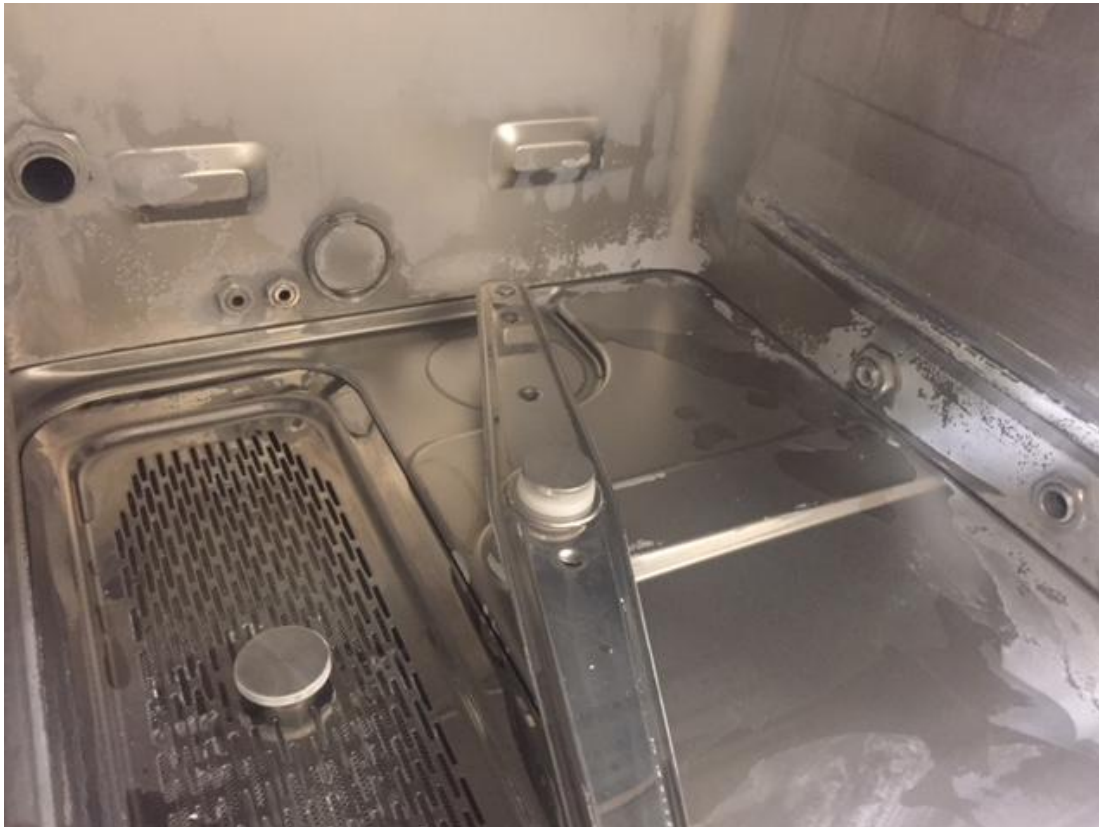
Figure 3: An example of lime scale build up within a washer disinfector
