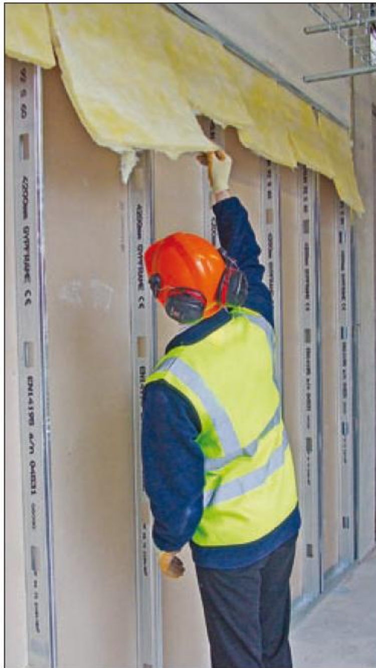
Site inspection (photograph courtesy of Sound Research Laboratories Ltd)
