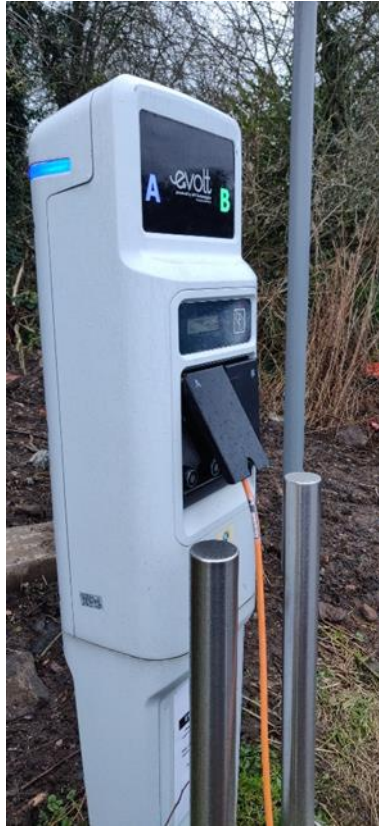
Figure 6: EV charging point with protective bollards
