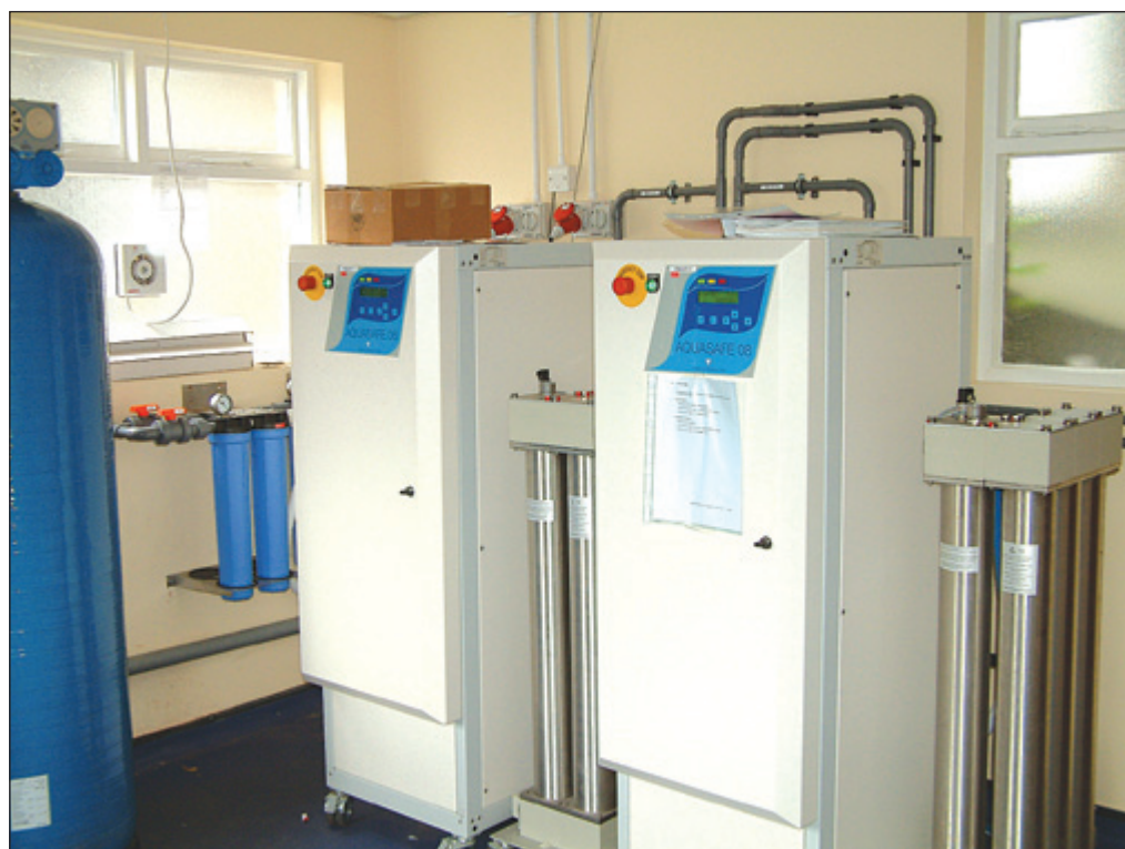
Water to be used for dialysis needs to be treated appropriately to remove impurities. For normal haemodialysis, water purity must meet the minimum standards for regular water quoted by the European Pharmacopoeia
