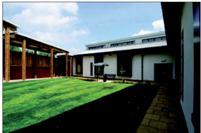
Use of shading to prevent solar gain. Photograph courtesy of Race Cottam Associates
