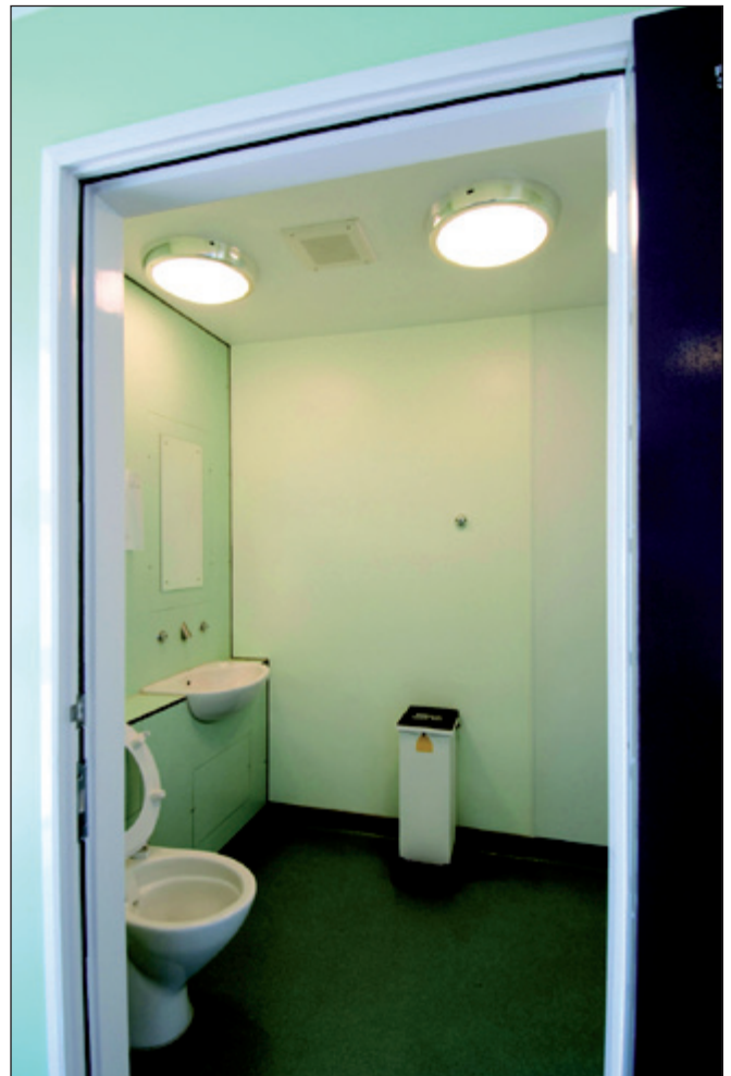
All fixtures and fittings should be anti-ligature
