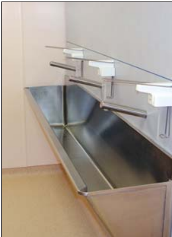
Figure 8 Scrub sink with non-touch taps
