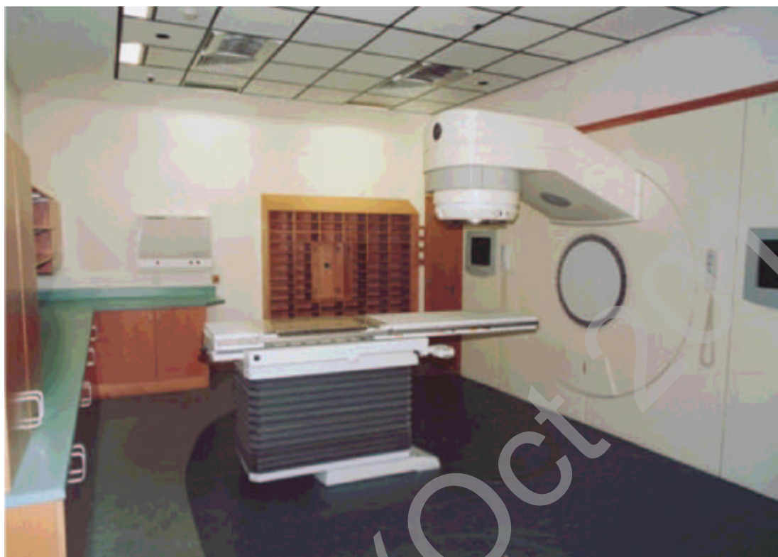
Linear accelerator treatment room where linac fascia panel is used to create a machine room
