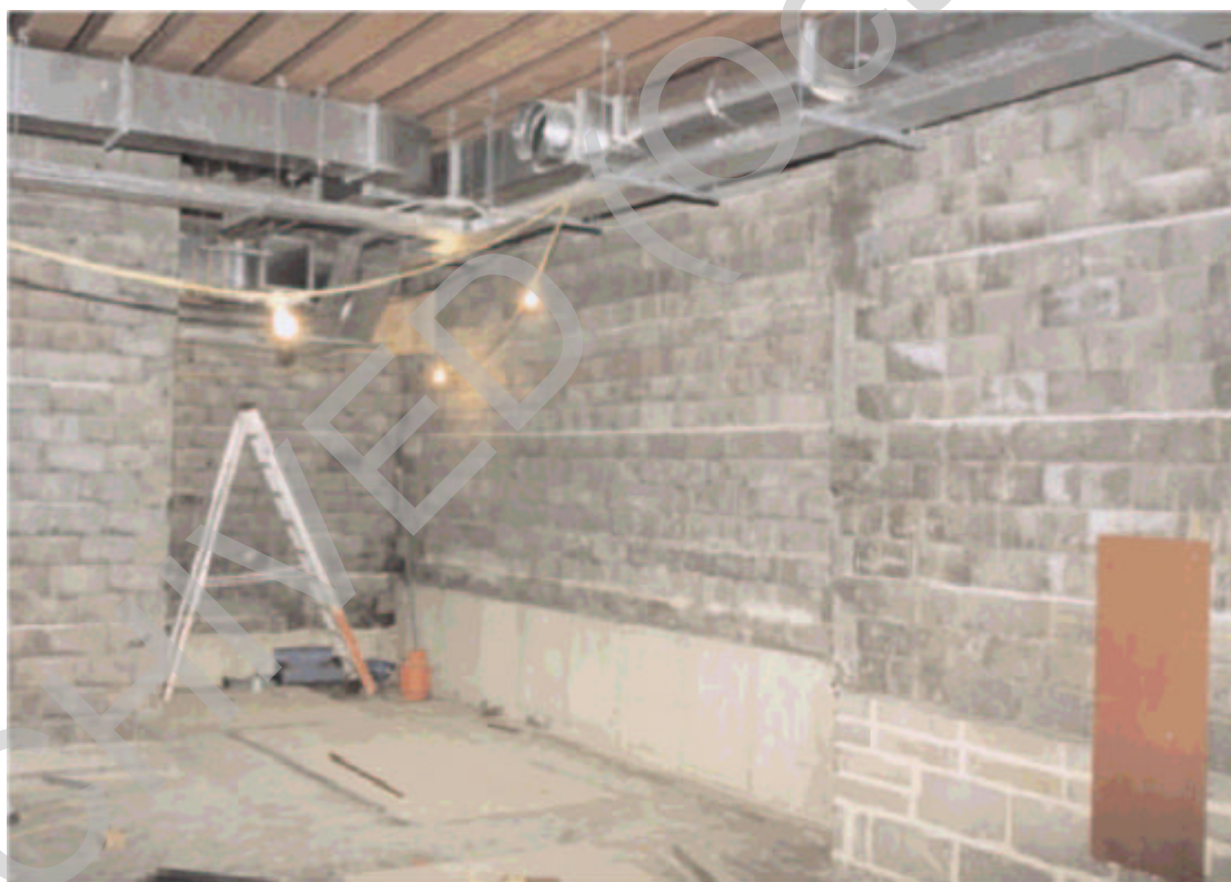
Internal view of linear accelerator bunker under construction using blocks of alternative shielding materials. Joints are formed using specialised proprietary mortar. Shows services entering from maze corridor and steel joists supporting roof structure.
