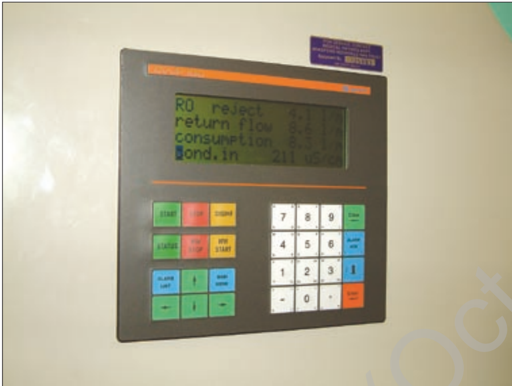
The water treatment plant conditions should be monitored by a plant status alarm panel providing visual or audible signals
