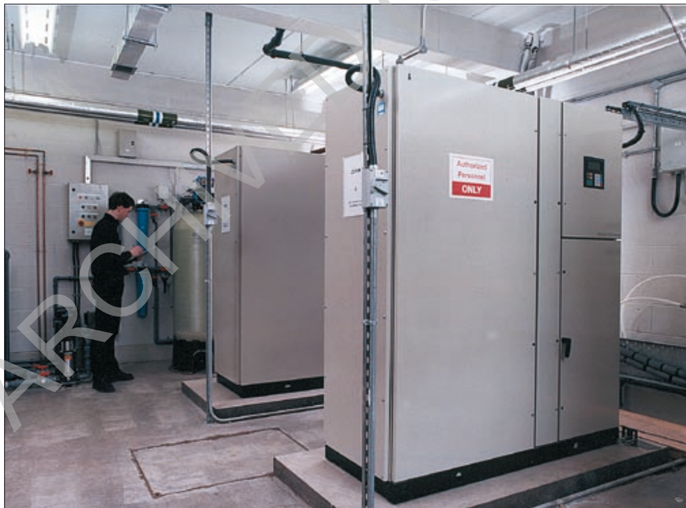
The quality of water that can be achieved with a central water-treatment plant is generally far higher than that which can be obtained from individual units. Courtesy of Esler Crawford Photography; reproduced by kind permission of Belfast City Hospitals Trust
