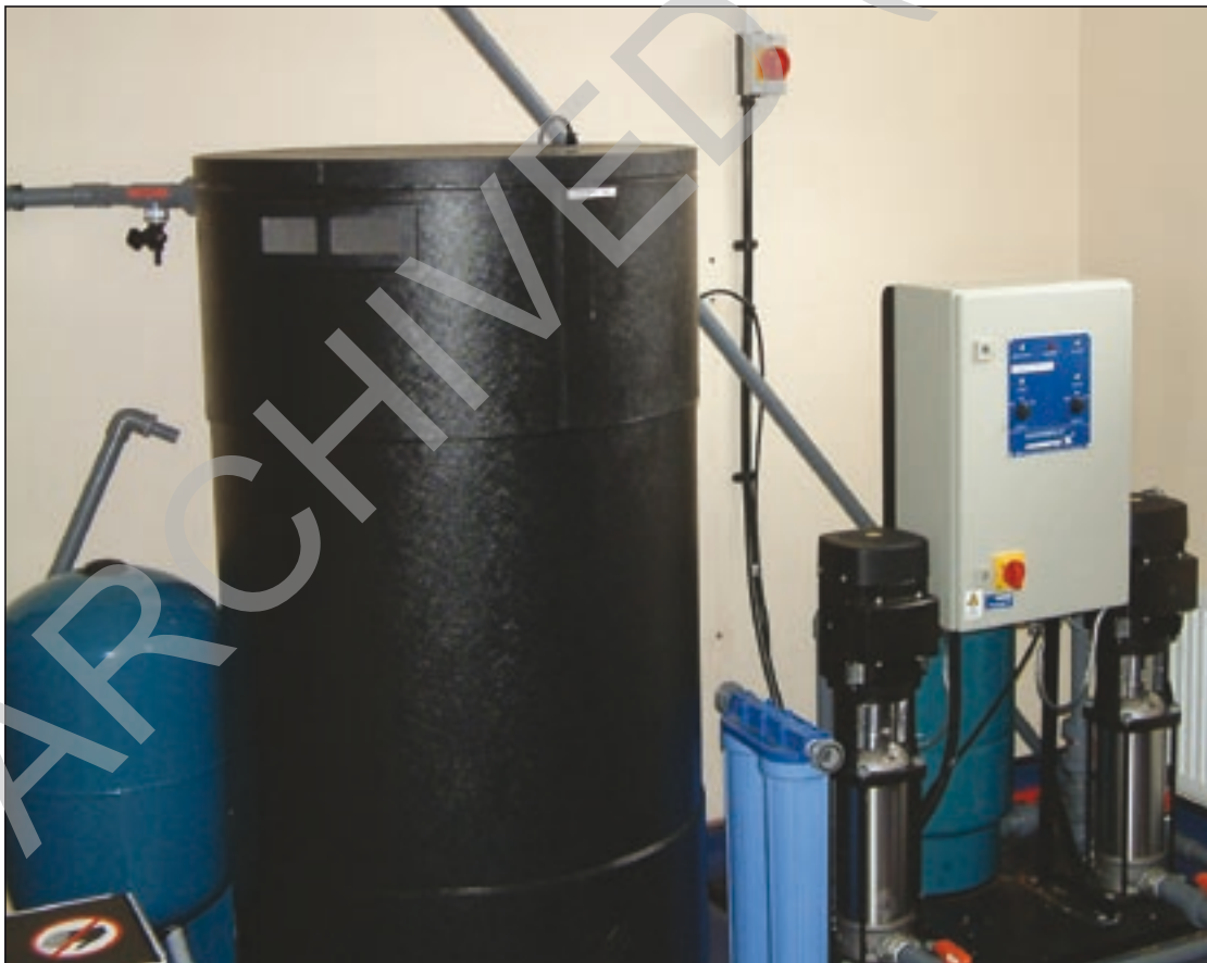
The water treatment plant should provide for total redundancy with dual softeners, circulating pumps, RO equipment and carbon filters
