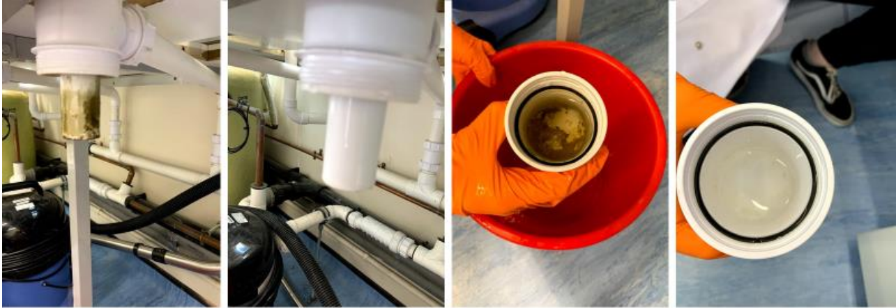
A. Base-draining sink: before and after treatment with a chlorine-based liquid disinfectant
