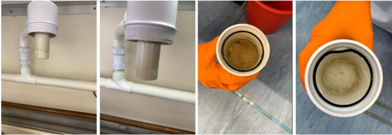
C. Rear-draining sink: before and after treatment with a peracetic acid-based liquid formulation
