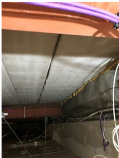
Figure 3.10 - RAAC plank cut short to sit on shelf angle has cracked bearing
