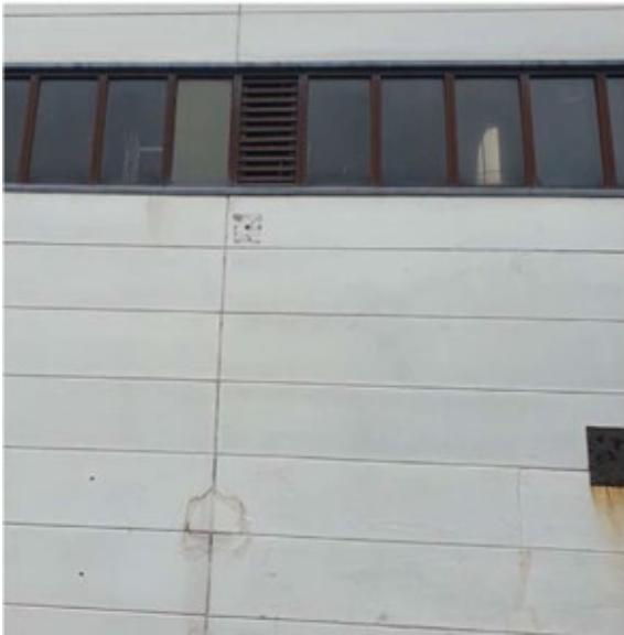
Figure 2.13 - Internal view of RAAC cladding panel
