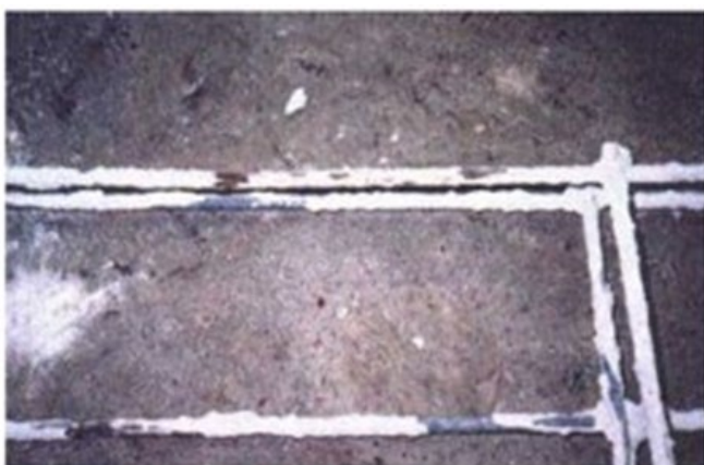
Figure 2.10 - Typical configuration of RAAC reinforcement (page 1, 'IP 10/96 - Reinforced Autoclaved Aerated concrete planks designed before 1980', BRE, December 1996)
