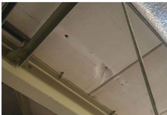
Figure 3.2 - Soffit spall
