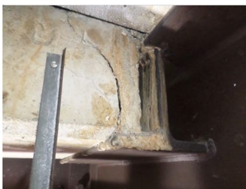
Figure 3.10 - RAAC plank cut short to sit on shelf angle has cracked bearing
