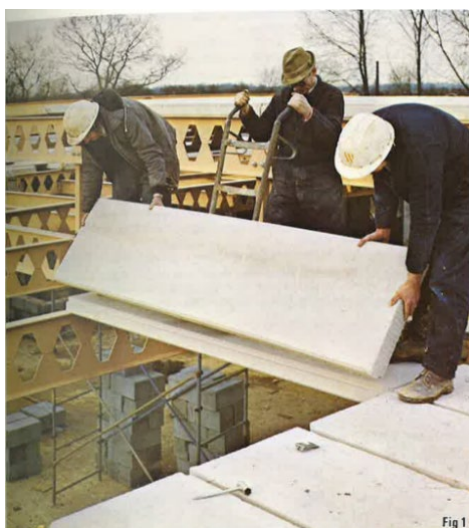
Figure 2.2 - Installation of a RAAC plank (page 1, 'Autoclaved Aerated Concrete Roof and Floor Units Handbook 2', Aerated Concrete Ltd, October 1977)
