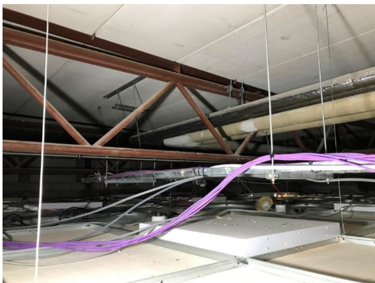
Figure 1.1 - RAAC planks supported on steel trusses
