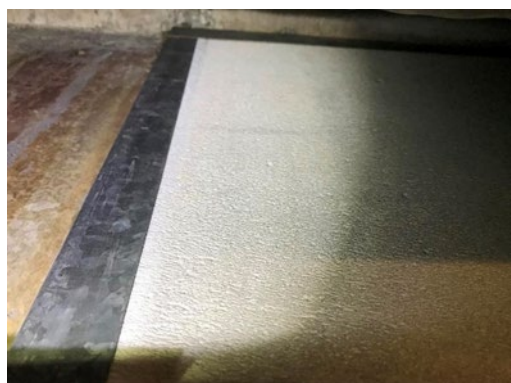
Figure 2.14 - Non-loadbearing RAAC partition
