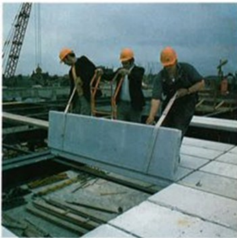
Figure 2.2 - Installation of a RAAC plank (page 1, 'Autoclaved Aerated Concrete Roof and Floor Units Handbook 2', Aerated Concrete Ltd, October 1977)
