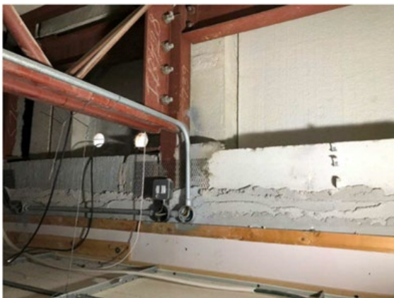
Figure 2.13 - Internal view of RAAC cladding panel
