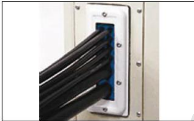
Figure 30: EMC compliance measures
